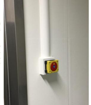
Again manufactured from extruded aluminium with specially treated steel boxes, BS4662 fixings or bespoke as required, these components offer equal resilience to the rigours of CL3+ cleaning and environment usage.
