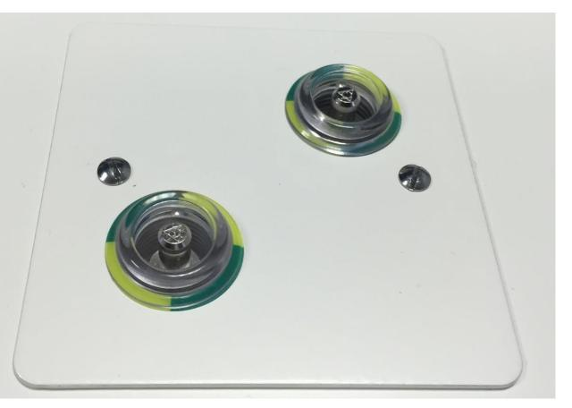
Supplementary equipotential bonding connection points for the connection of ME equipment shall be provided in each medical location, as follows:
