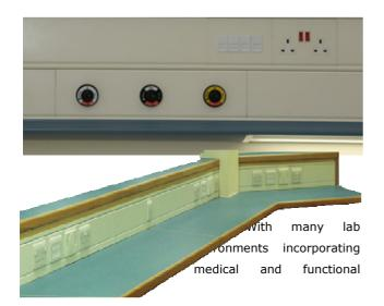
gases a range of gas terminal units and valves by leading industry providers can be catered for. Located in a separate chamber for both gases and liquids as required, the requirements of ISO 11197 are fully embraced.
